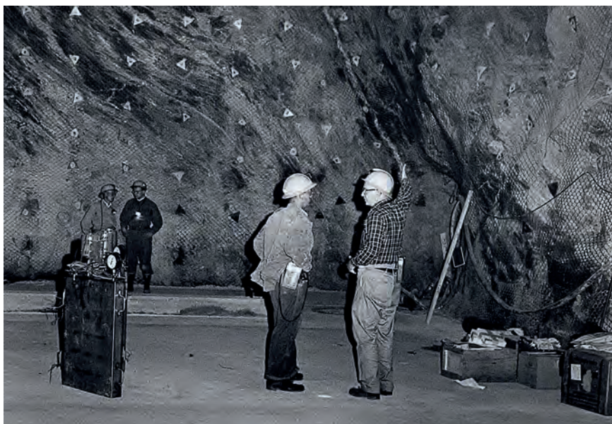
A historic view of the Davis Cavern that hosted Ray Davis's Nobel Prize-winning solar neutrino experiment. The cavern has since been expanded and its walls have been coated with shotcrete, a type of spray-on concrete, to accommodate research on dark matter. Photo Credit: Anna Davis, Sanford Underground Research Facility.
